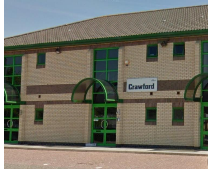
NB. PHOTO OF SIMILAR ADJACENT BUILDING
